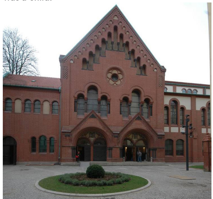
Exterior of the renovated Rykestrasse Synagogue. (The Center for Jewish Art Collection; available via the National Library of Israel Digital Collection)
